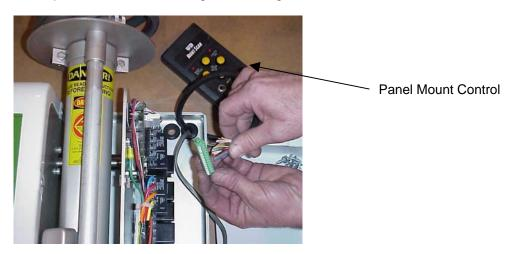
2. Strip wire ends and connect per wiring diagram in Appendix B.
