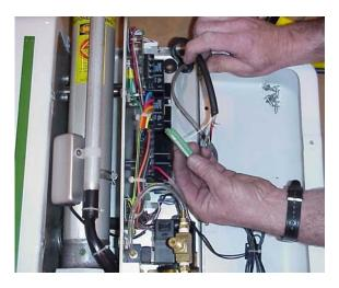
4. Strip wire ends and connect per wiring diagram in Appendix B.
